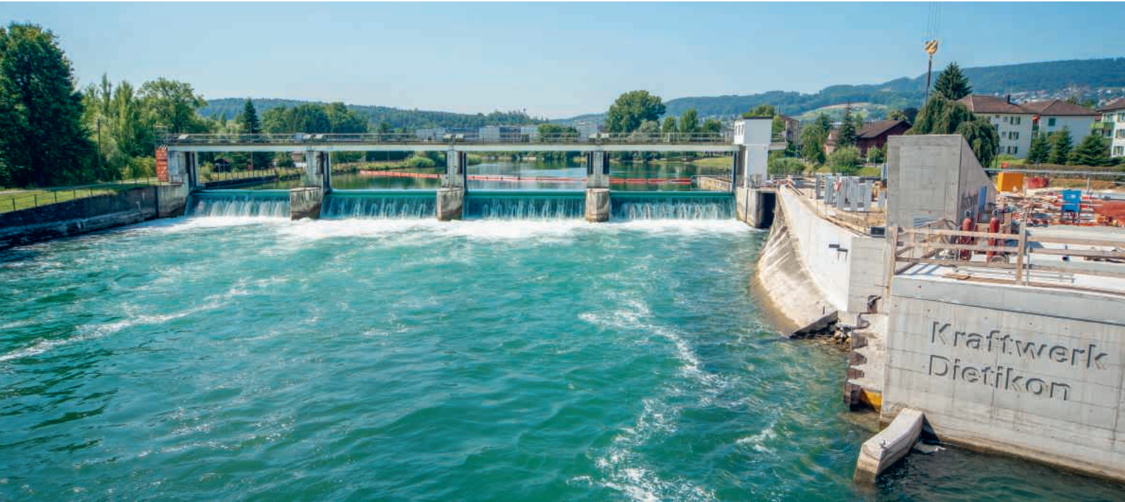
EKZ weir power station, Dietikon (ZH)
