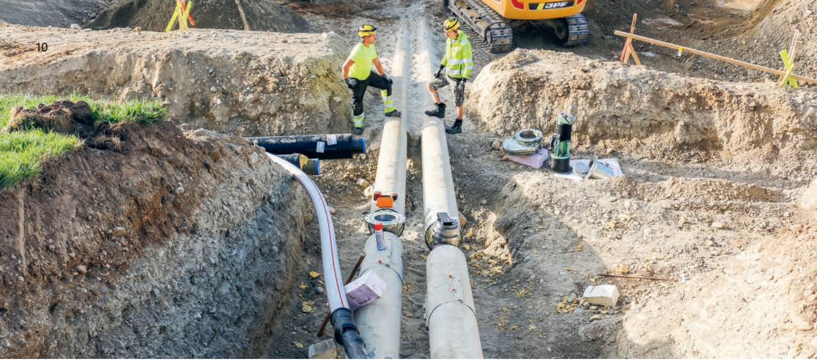
Line stopping service for PREMANT pipe in Posieux, Switzerland
