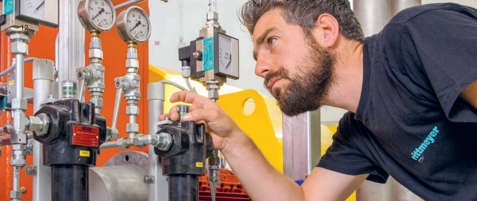
Commissioning of a hydropower plant
