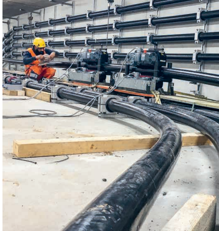
Cable laying 380kV Gäbihübel in Riniken, Switzerland
