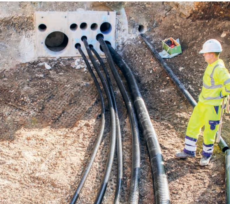
CALPEX and COOLFLEX installation in Baden, Switzerland
