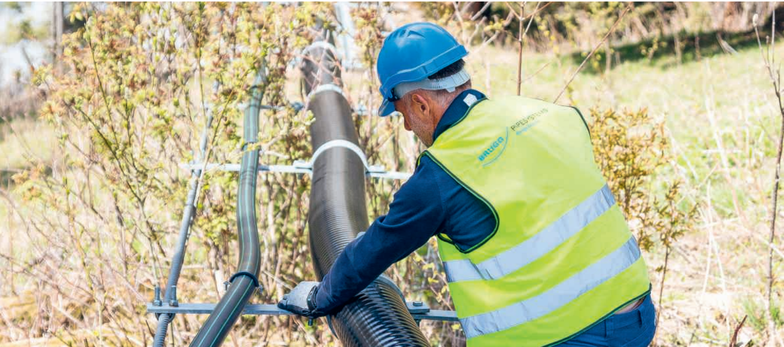
EIGERFLEX pipe with integrated frost-protection strip in Kiental, Switzerland
