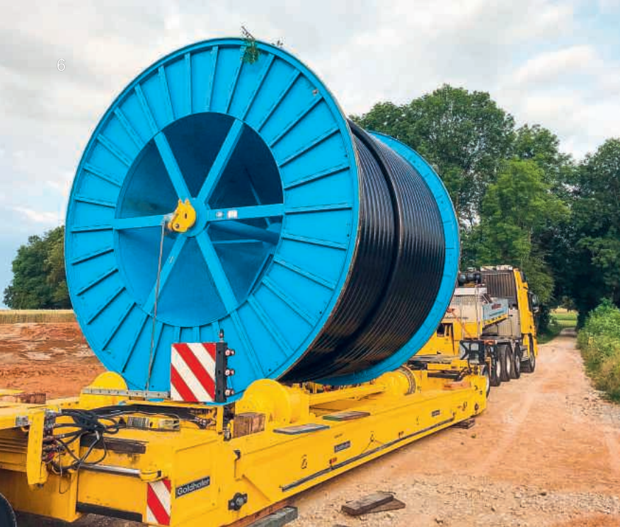
Cable laying 380kV Gäbihübel in Riniken, Switzerland
