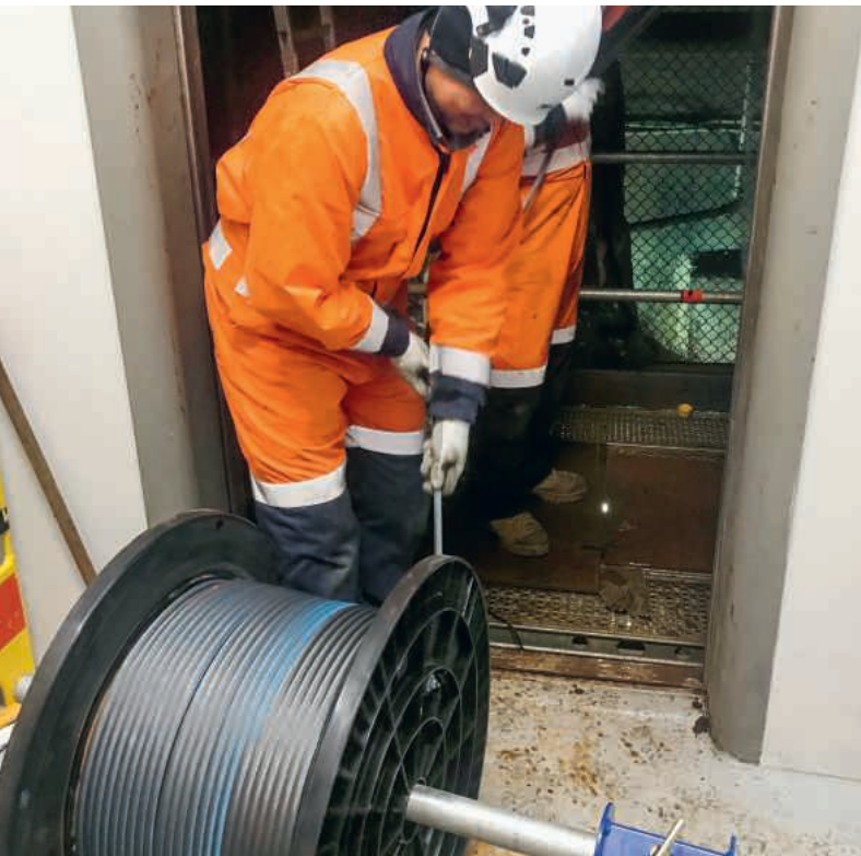
Installation of a BRUGG elevator rope
