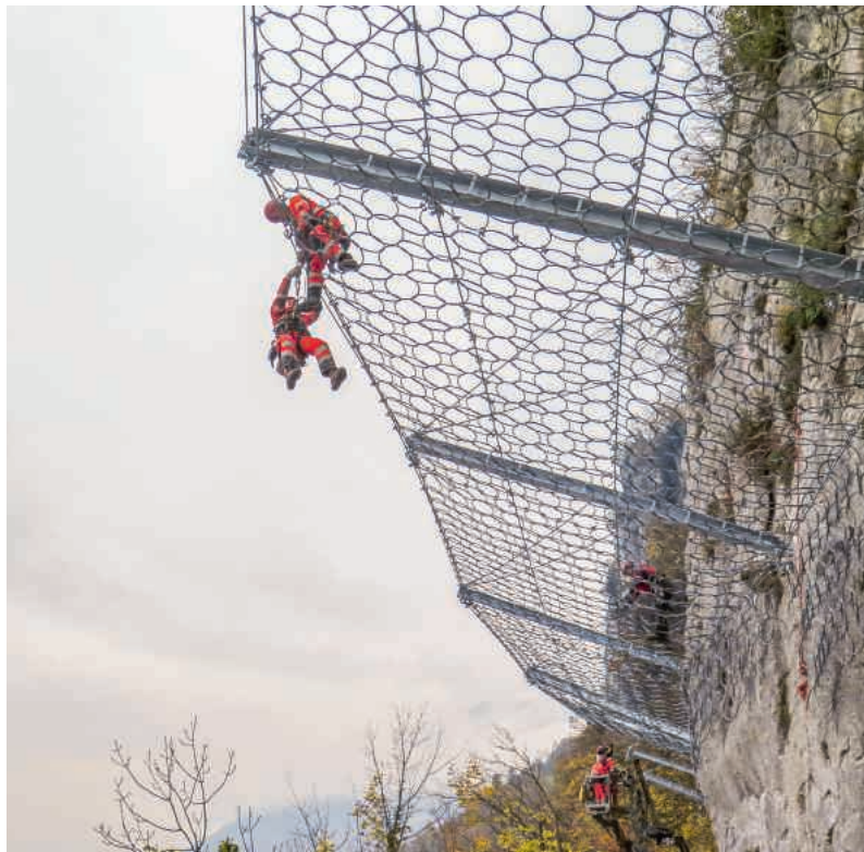
Installation of a Geobrug rockfall protection barrier
