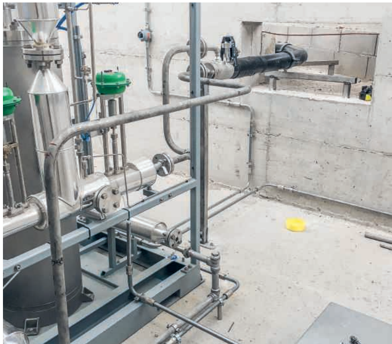
Connecting a service station with FLEXWELL-LNG in Perugia, Italy
